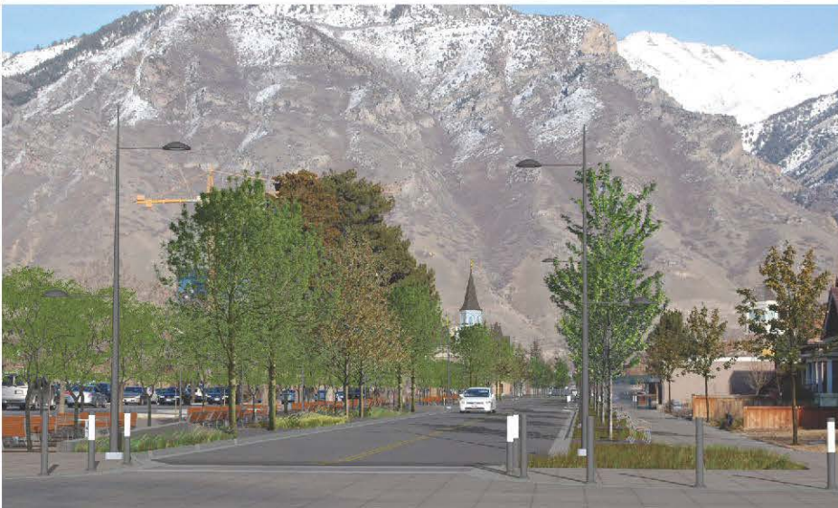
After street reconstruction
