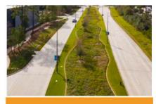
Bioswales: Vegetated channels or swales are designed to direct and slow down stormwater runoff, filter pollutants, and allow for water infiltration rather than directing water to underground pipes along roadsides or parking lots.
