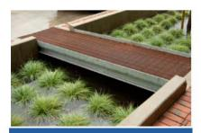
Rain Gardens: Small depressions, planters, or recessed gardens capture and absorb water to allow infiltration into the ground rather than flowing directly into storm drains.
